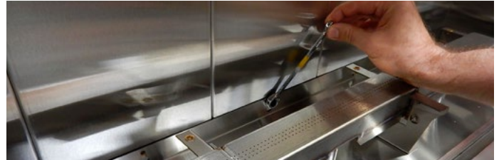
Figure 42 Loosening air baffle bolts
