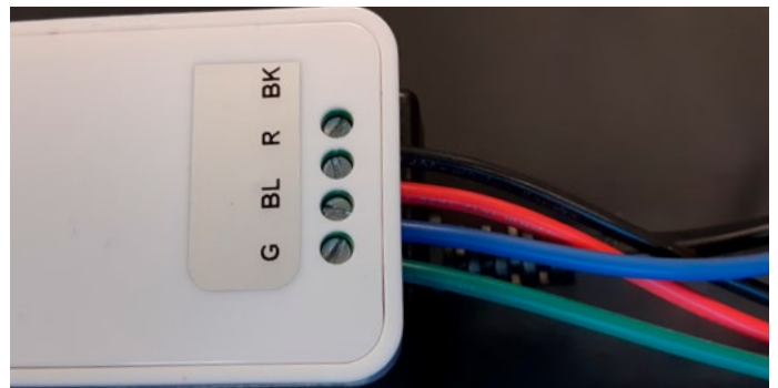
Figure 35 Wiring the LED receiver
