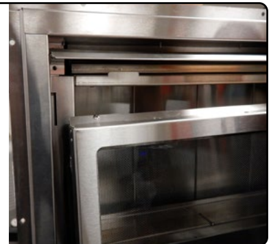
Figure 61 Completing removal of the door
