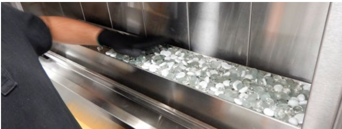
Figure 64 Installation of the firestones. (Ensure ONLY one layer of firestones cover the burner surface).
