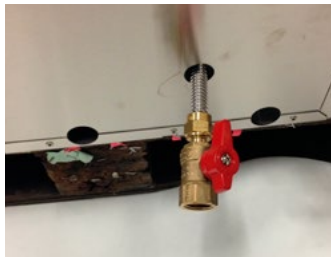
Figure 12 Gas connection
