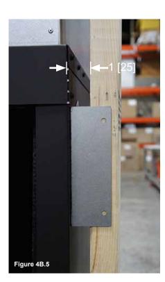
The nailing tabs will ensure the 1" [25] minimum clearance is kept to combustible framing.
