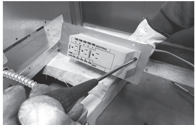
Figure 8.6 Junction Box Removal
