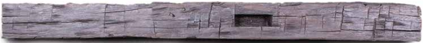
Hewn Mortise Beam
