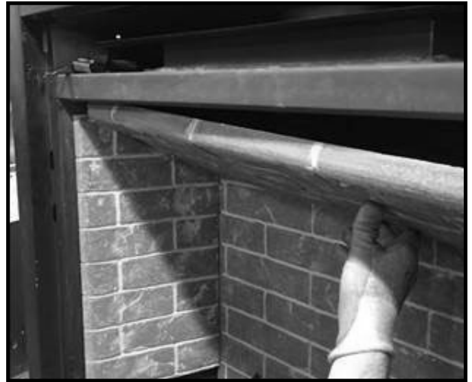
Figure 11.4 Install Top Refractory Panel
