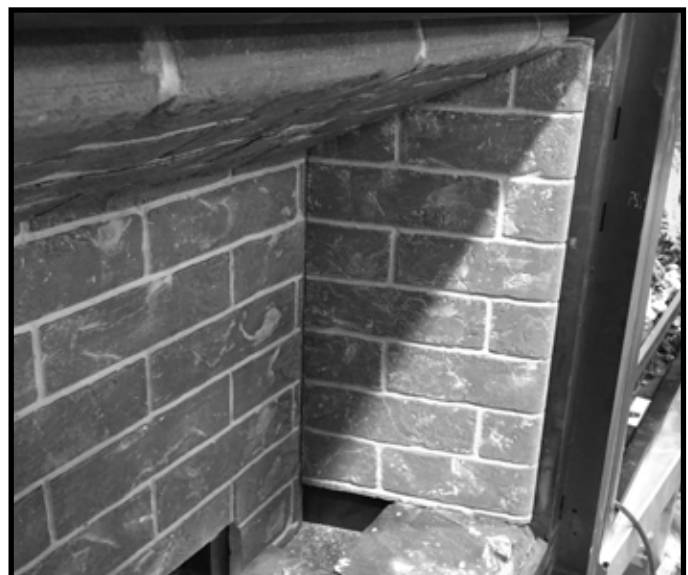
Figure 11.6 Right Refractory Panel Installed
