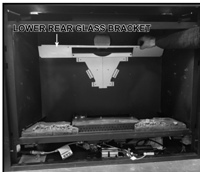
Figure 11.8 Removing Lower Rear Glass Bracket
